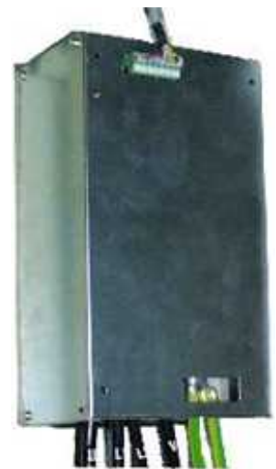
Fig. 11-4 LE200-Thyristor power stage with cover
