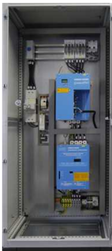
Fig. 2-20 Control cabinet with GeniusHWI master/slave
