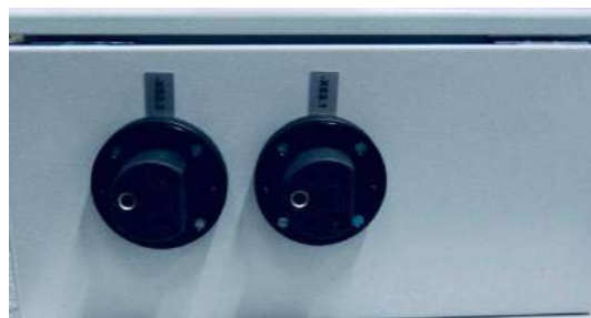
Fig. 6-6 LVMU power distribution and measurement signal switchover
